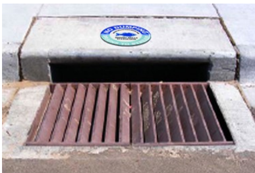
Combo curb/ grate inlet
